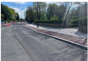
The outbound road has been reconstructed along this section with the final surfacing yet to be applied.
